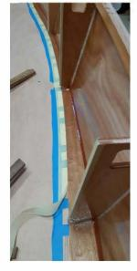
I decided to epoxy the inside of the hull walls before fixing the side tank Panels as less room behind once in position. All taped up and ready to rumble. (Epoxy). Side Panel fixed and filleted. Side tank panel to Transom showing the Bung hole in the rear air tight tank.
