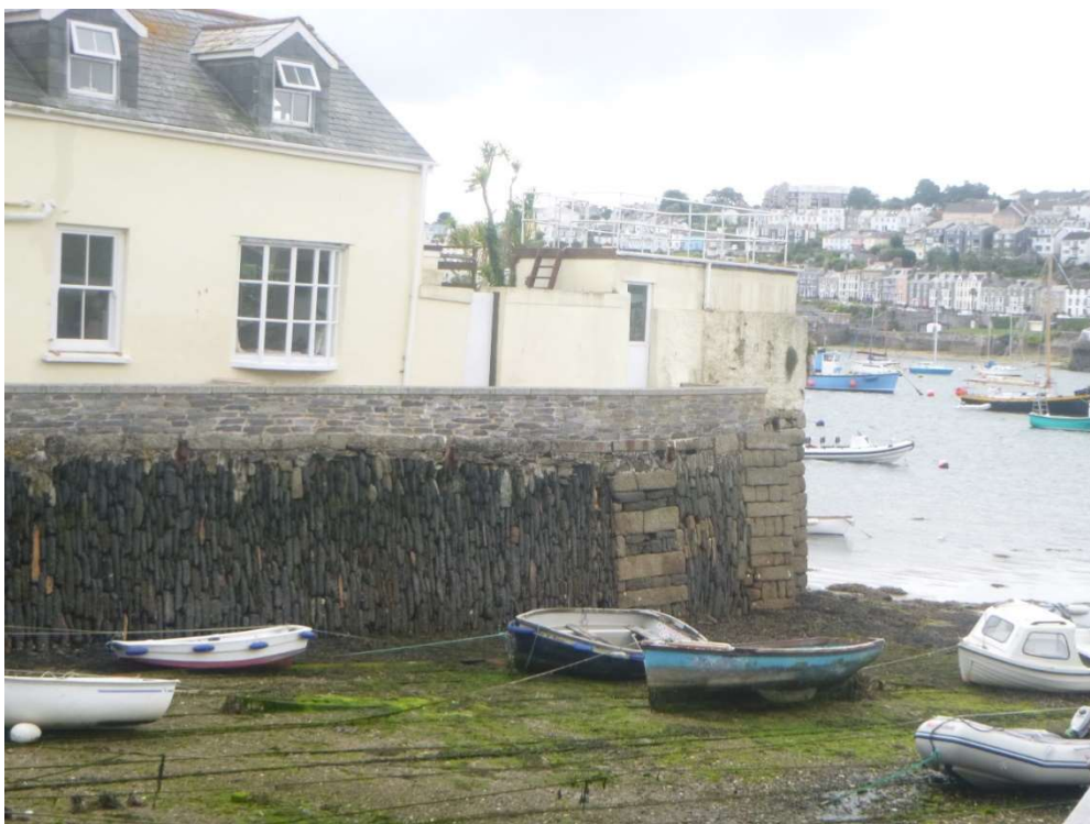
Flushing harbour was built by a Dutch team from the town of the same name, and has characteristic vertical slabs
